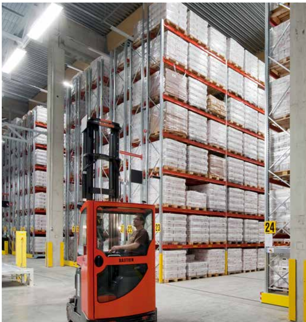
Mobile pallet racking (MOVO) | 21,500 pallet positions
